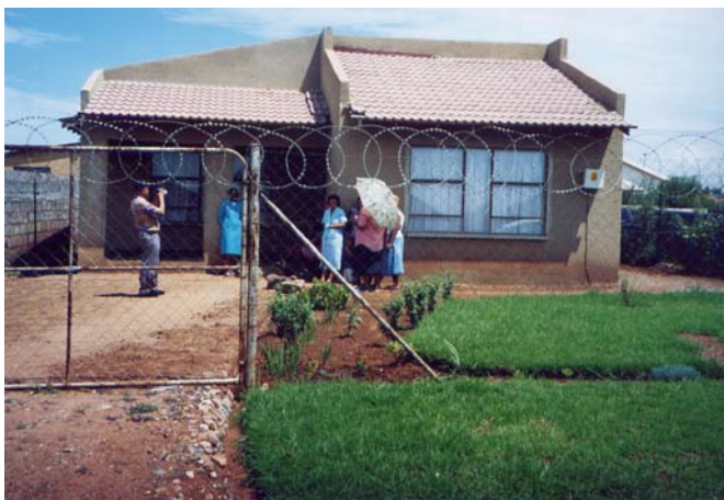
A significantly improved RDP house in Vosloorus, Gauteng.
